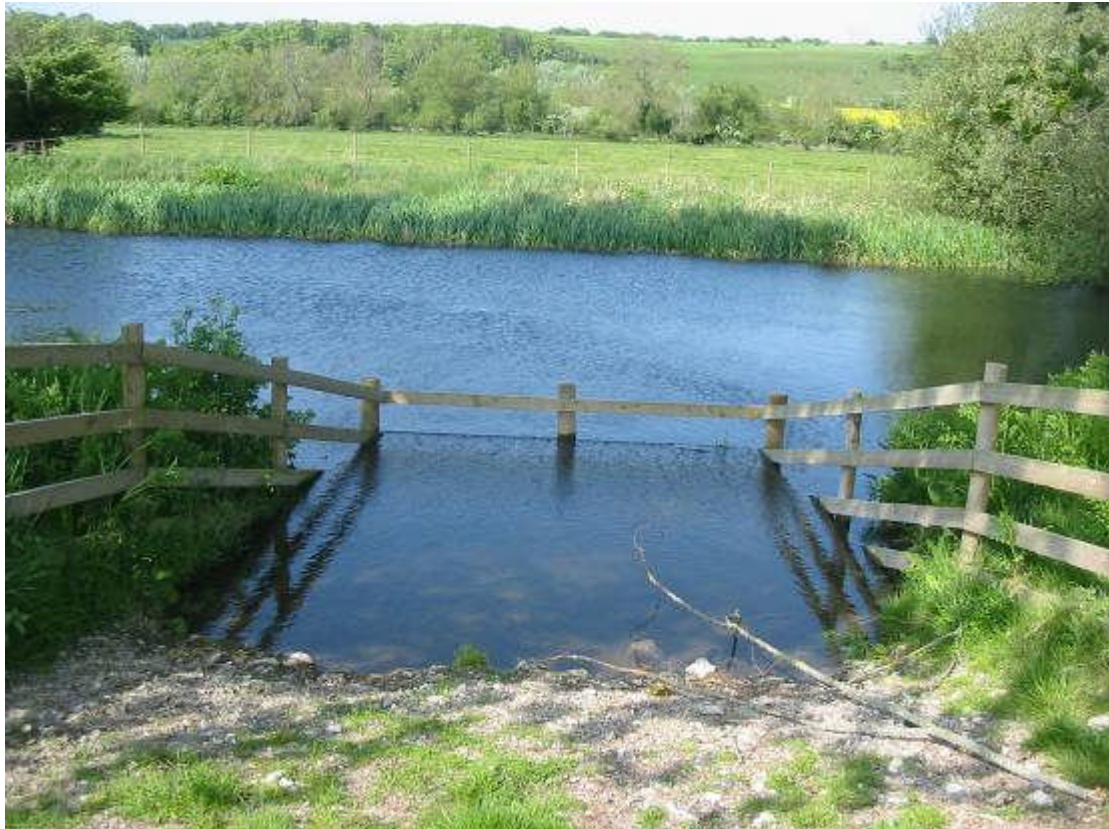
Well designed cattle drinking area
